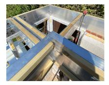
Sections couple together easily using high tensile bolts and solid 12mm gauge aluminium plates
