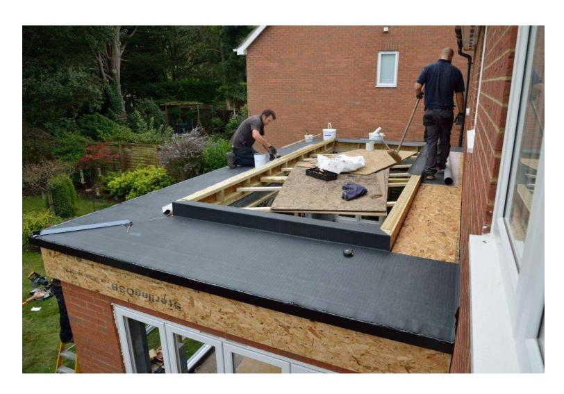
Once insulation and decking boards have been fixed into place the perimeter roof section can have the specified covering applied
