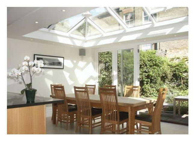
**iX250** is a bespoke manufactured aluminium deck system that is designed specifically to support a glazed lantern within a flat roof area. The main benefits being that all the sections have been pre-fabricated which means site is easily accessible and a speedy on site build time is ensured. With all builds there is also an option for 100mm or 125mm insulation & external plywood to be supplied pre machined and a complete gutter & fascia pack if required.
